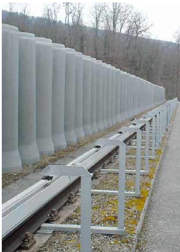
SACL system application
